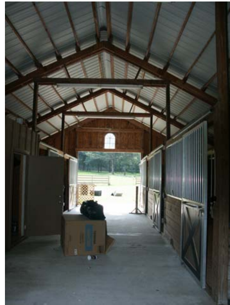
Interior of Barn
