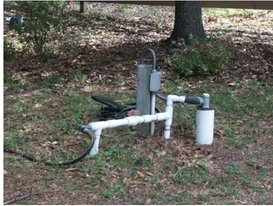
Well at NE corner of house
