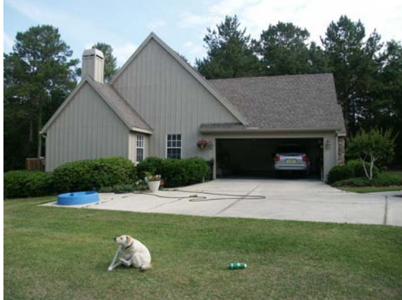
Concrete Drive on south side of house
