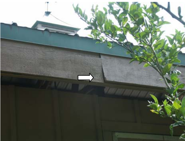
Fascia at south side of barn
