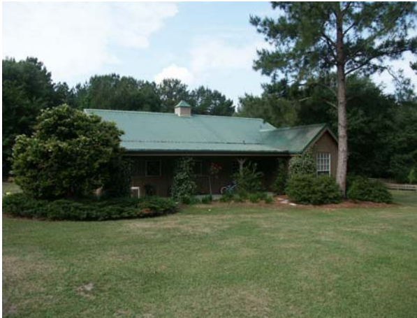
Front (North) view of Barn/Apartment
