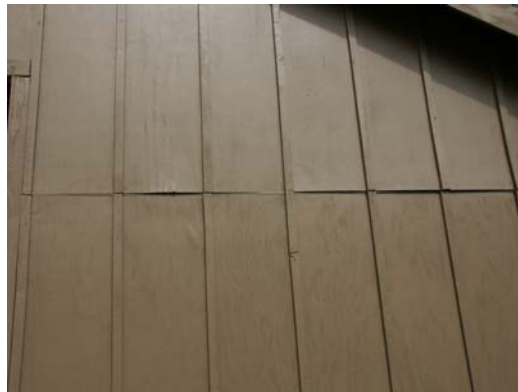
Siding at barn
